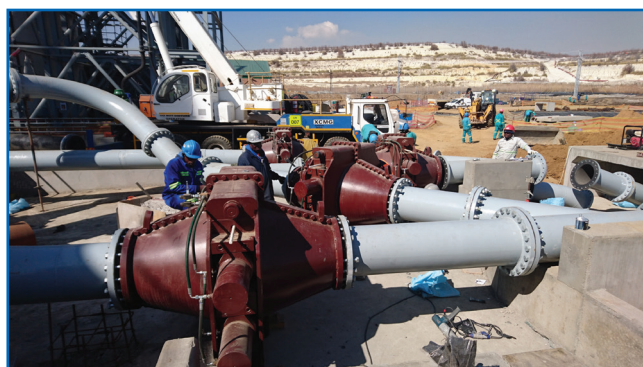
450mm Corflex Pinch Valves at Evander
